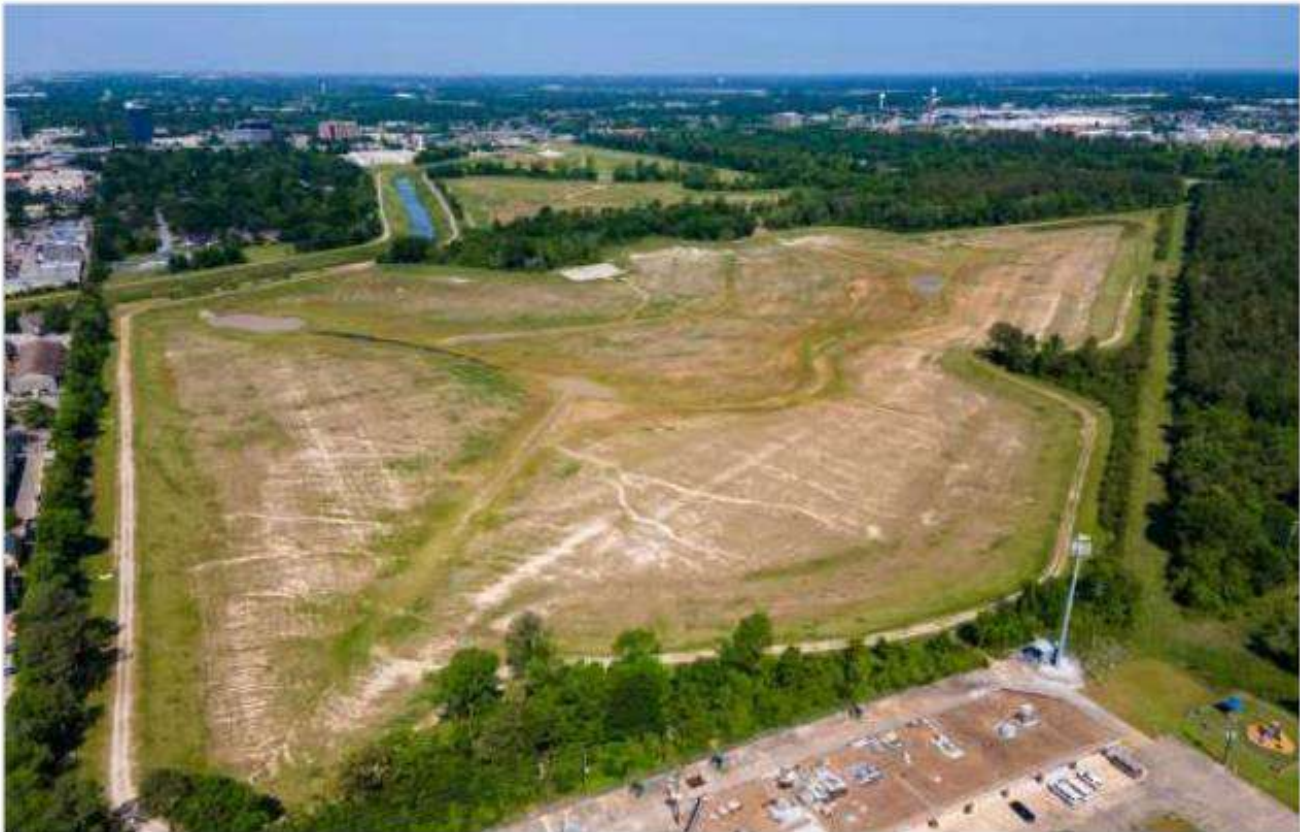
Glen Forest Stormwater Detention Basin (P500-08-00)
