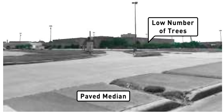
Figure 2.31 Street view of Greens Road facing Greenspoint Mall, one of the hottest roads in North Houston. The lack of trees and heavily paved areas cause this area to become very hot.
