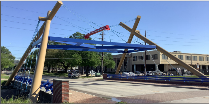
New paint on Greenspoint Bridge
