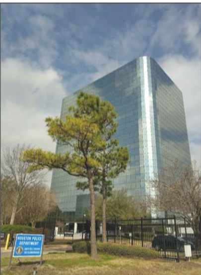
New HPD North Belt Division headquarters
